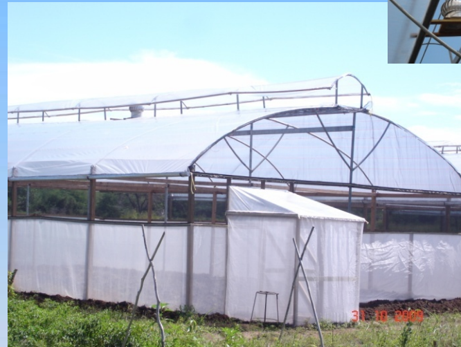
Center vent, cooling fan, sidewalls with combination of antiviral mesh and shade cloth
