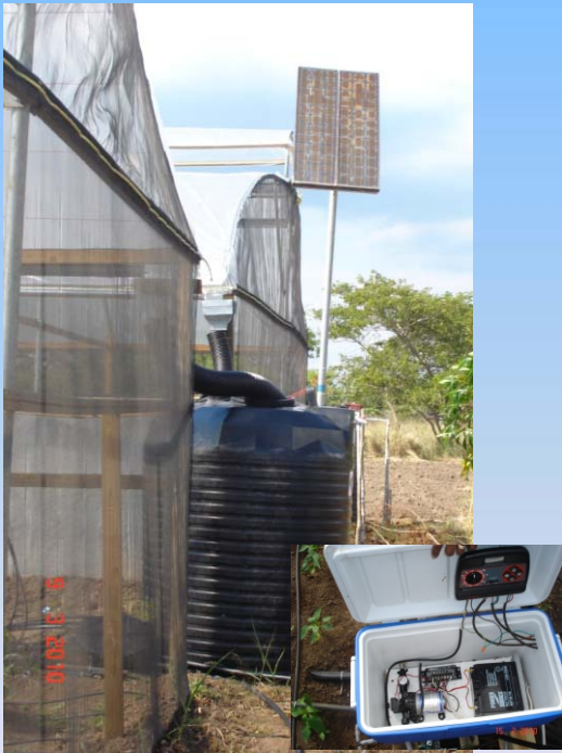
Fertigation system is solar-powered by photovoltaic cells
